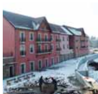
Montcenis Nursing Home. Over 6100 m 2 and 85 rooms. Saône et Loire, France. ECO-G
