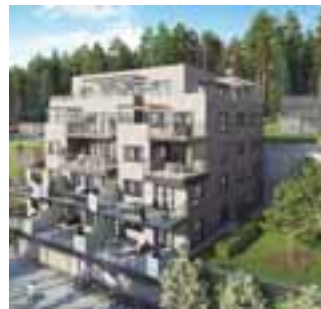
New condominium. Bergås Terrasse complex. Drammen, Norway. ECOi / Aquarea
