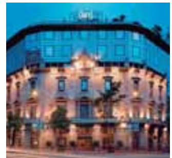
Hotel refurbishment. Hotel Claris 5 * Barcelona, Spain. ECOi
